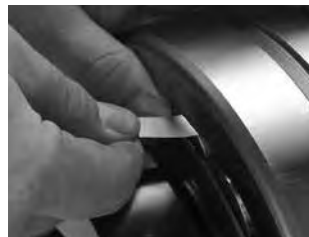
Fig. 91. Measure RIC before installation.
